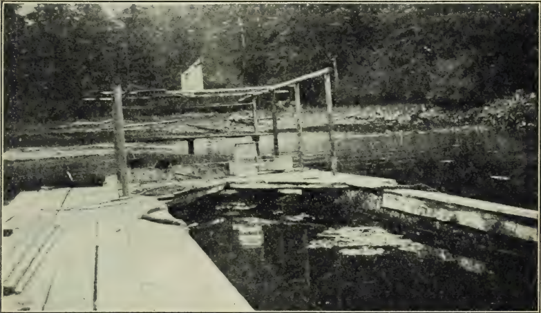
FIG. 8.—A floating dock of the type illustrated can be built easily and cheaply and is a great convenience in landing supplies and tying up a boat in the harbor
